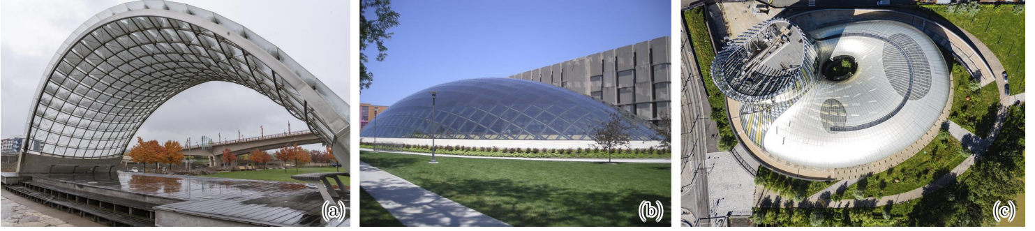
Figure 2: Planar beams in architectural structures. (a) Schubert Club Band Shell, designed by James Carpenter Design Associates (image from flickr.com photographed by Tony Webster under CC BY-SA 2.0). (b) Joe and Rika Mansueto Library, designed by Murphy/Jahn in 2011 (image from wikimedia.org photographed by Michael Barera under CC BY-SA 4.0). (c) La Cité du Vin in Bordeaux, designed by Anouk Legendre and Nicholas Desmazières of XTU Agency in 2016 (image from flickr.com photographed by Adrien Sifre under CC BY-NC-ND 2.0).
