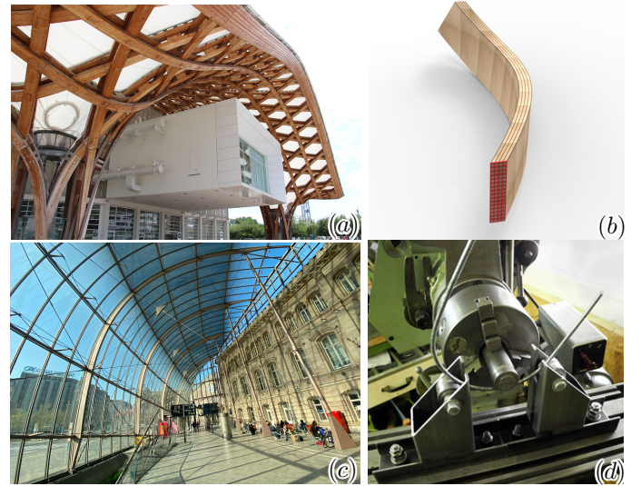
Figure 3: (a) Non-planar timber beams, such as the ones of the Centre Pompidou Metz (designed by Shigeru Ban), are curved in two directions (image from flickr.com photographed by Fred Romero under CC BY 2.0). (b) Hence, when fabricated by gluing laminated timber, the wooden strips must be subdivided into an array of rods (highlighted in red). (c) In the gridshell structure of the Strasbourg train station (designed by AREP), the planar beams are made from steel and can easily be reinforced by “bike-wheel” cable diaphragms. (d) A roller bender bends the steel with three rollers in a plane (image from flickr.com photographed by Fred Romero under CC BY-ND 2.0).
